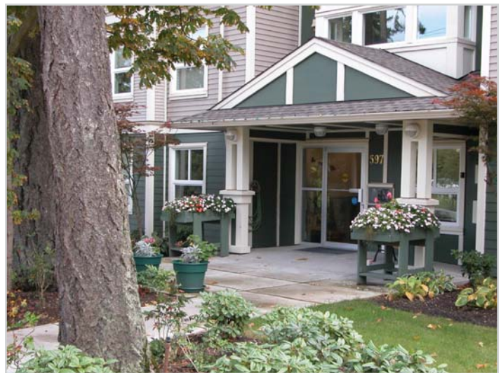
Figure 1 The front entrance at Fairway Woods
